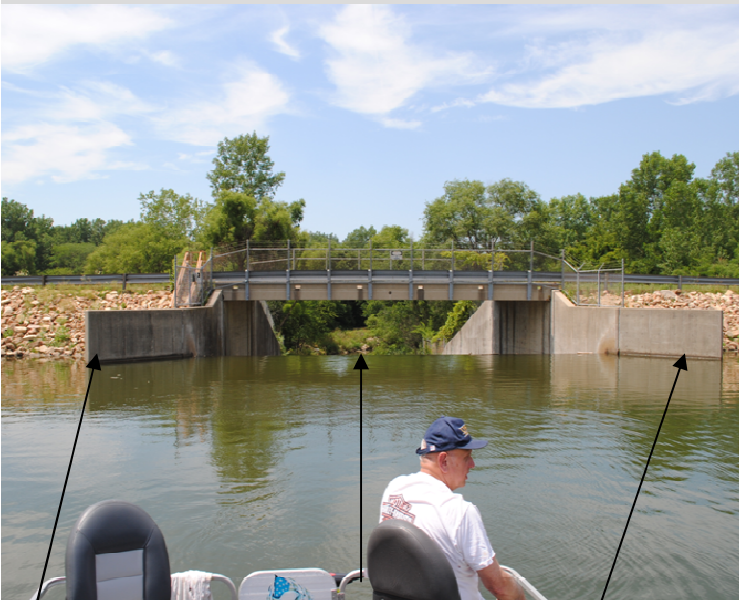
5’ Reading out from dam
